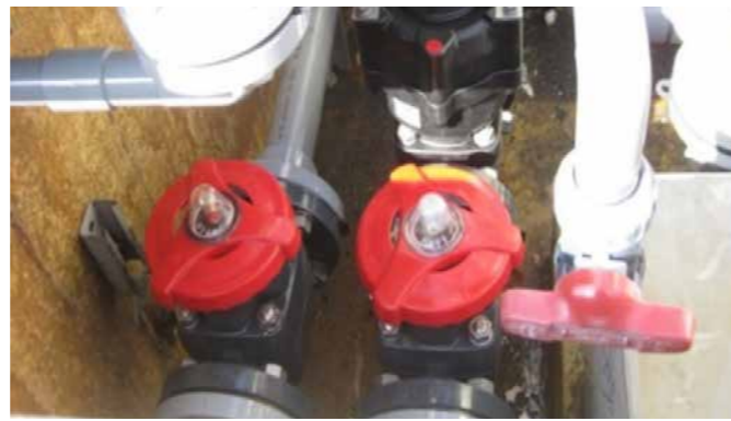
Chemical leakage countermeasures, emergency shutoff valve anchor installation
