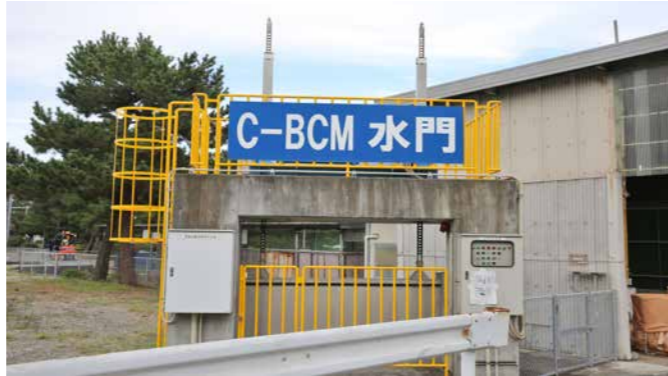
Sluice gates for tsunami countermeasures
