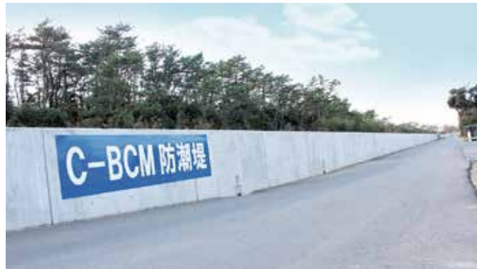
Breakwaters for tsunami countermeasure
